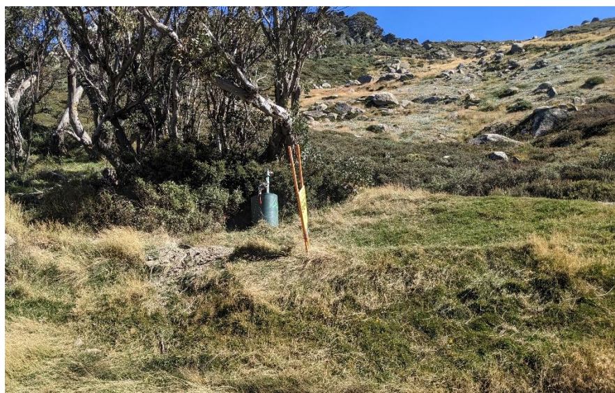
Figure 9: Photo of existing manual hydrant to be upgraded to a double hydrant
