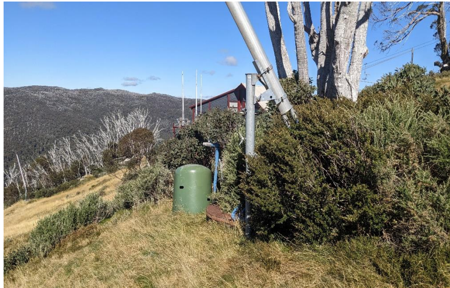
Figure 13: Photo of existing lance gun to be replaced with new lance gun and pit
